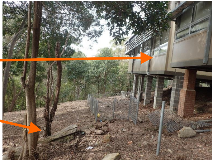
Photograph 05: View northeast of the existing APZ
