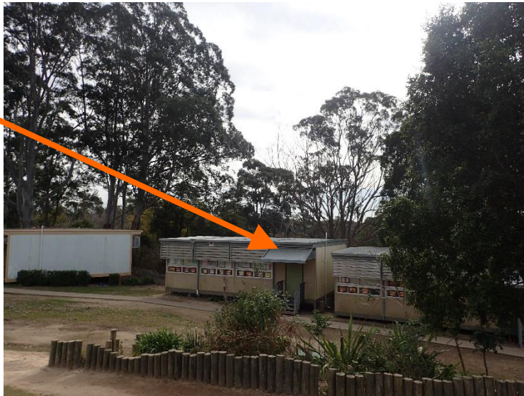
Photograph 01: View northwest from within the subject site toward existing demountable buildings (To be demolished)
